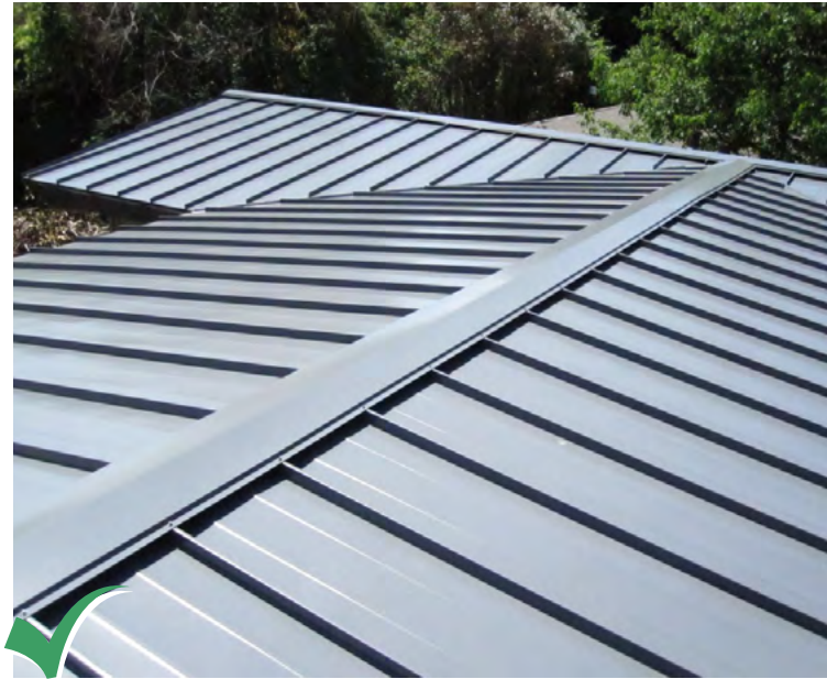
A standing seam metal roof will make a great, long lasting replacement.
