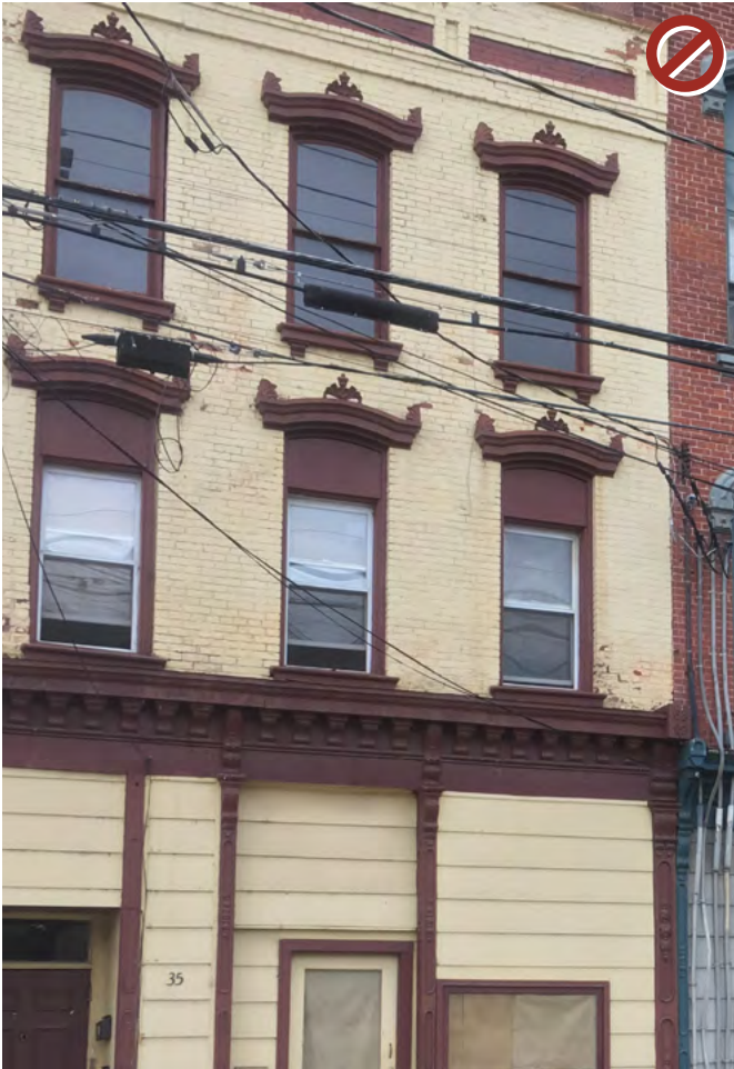
Do not fill in ground level storefronts with residential windows, doors, or siding.
