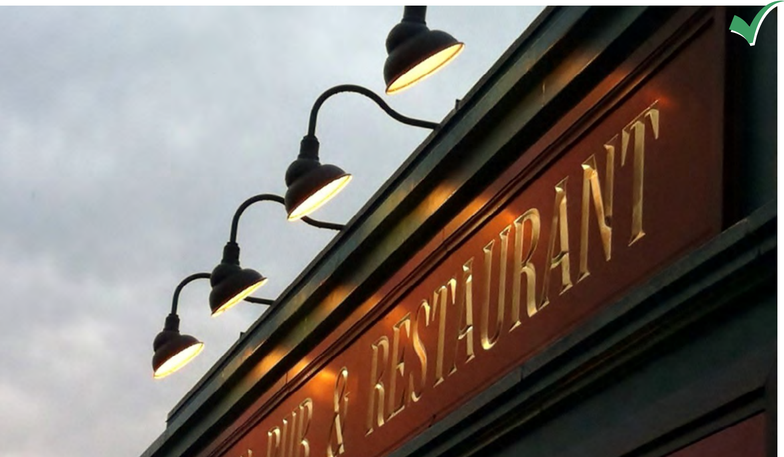
Space fixtures apart to create an even level of lighting across a signboard.
