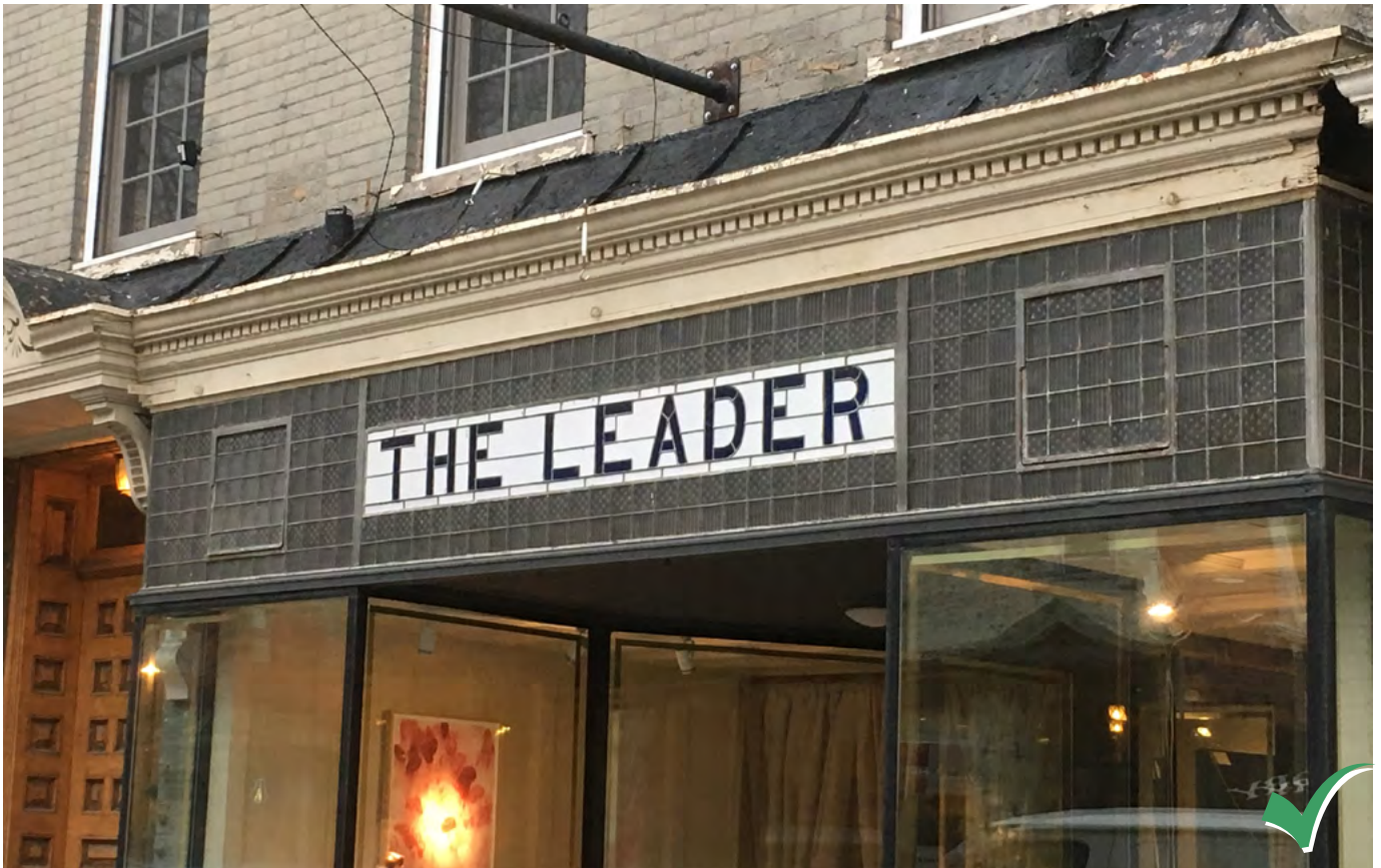
Restored transom window zones can be utilized as a unique signage opportunity.
