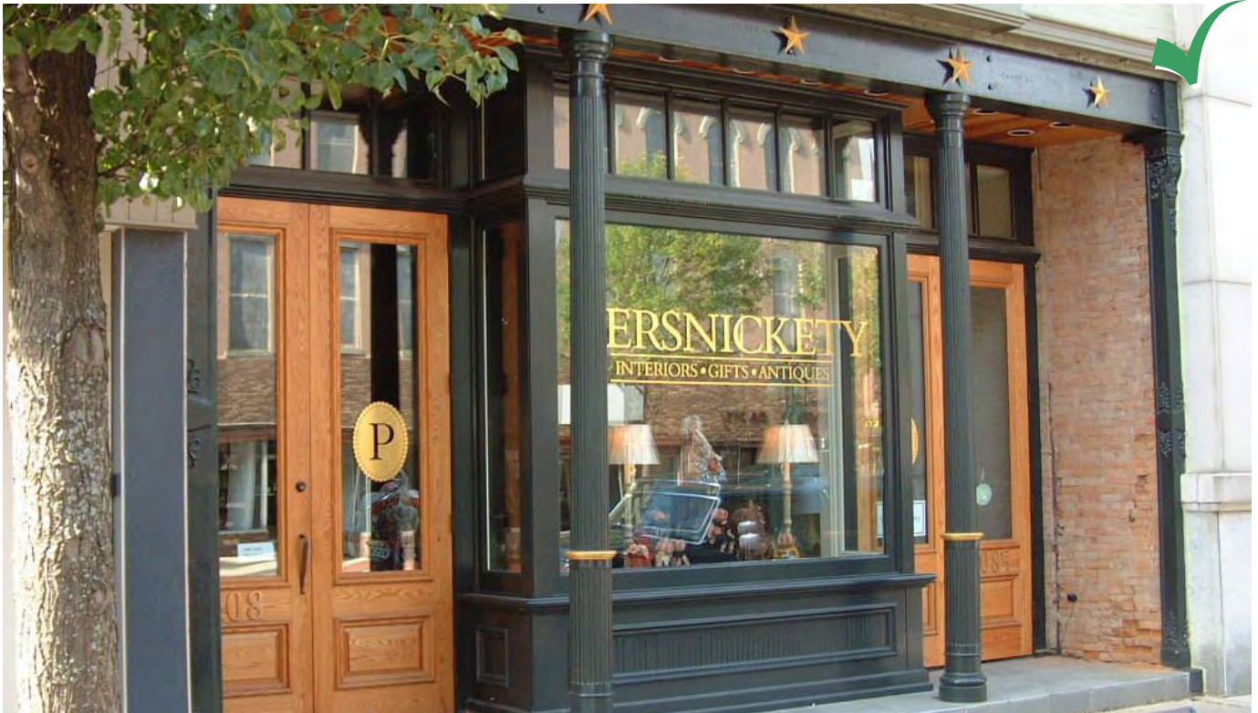
Use and maintain wood details when appropriate, such as at storefronts, windows, and doors.
