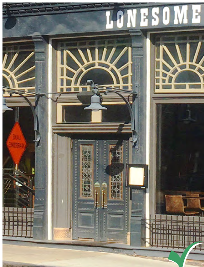
Restore historic detailing on and around doors and openings. Use color to highlight detail.
