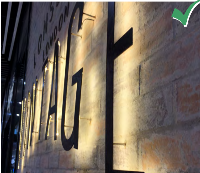
Letters can be backlit if they are illuminated only on their exterior.
