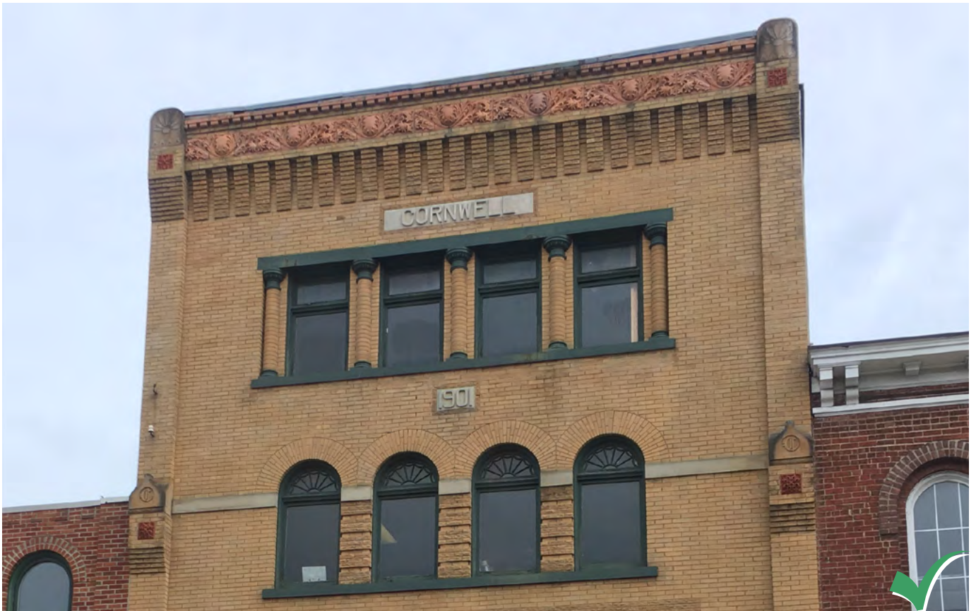
Restore and maintain historic masonry detailing and unique window features.
