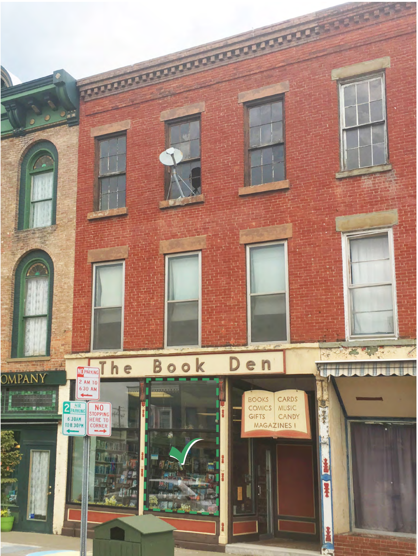
New storefront replacement windows should be sized to match existing openings and have similar sash profiles to the original windows if possible.
