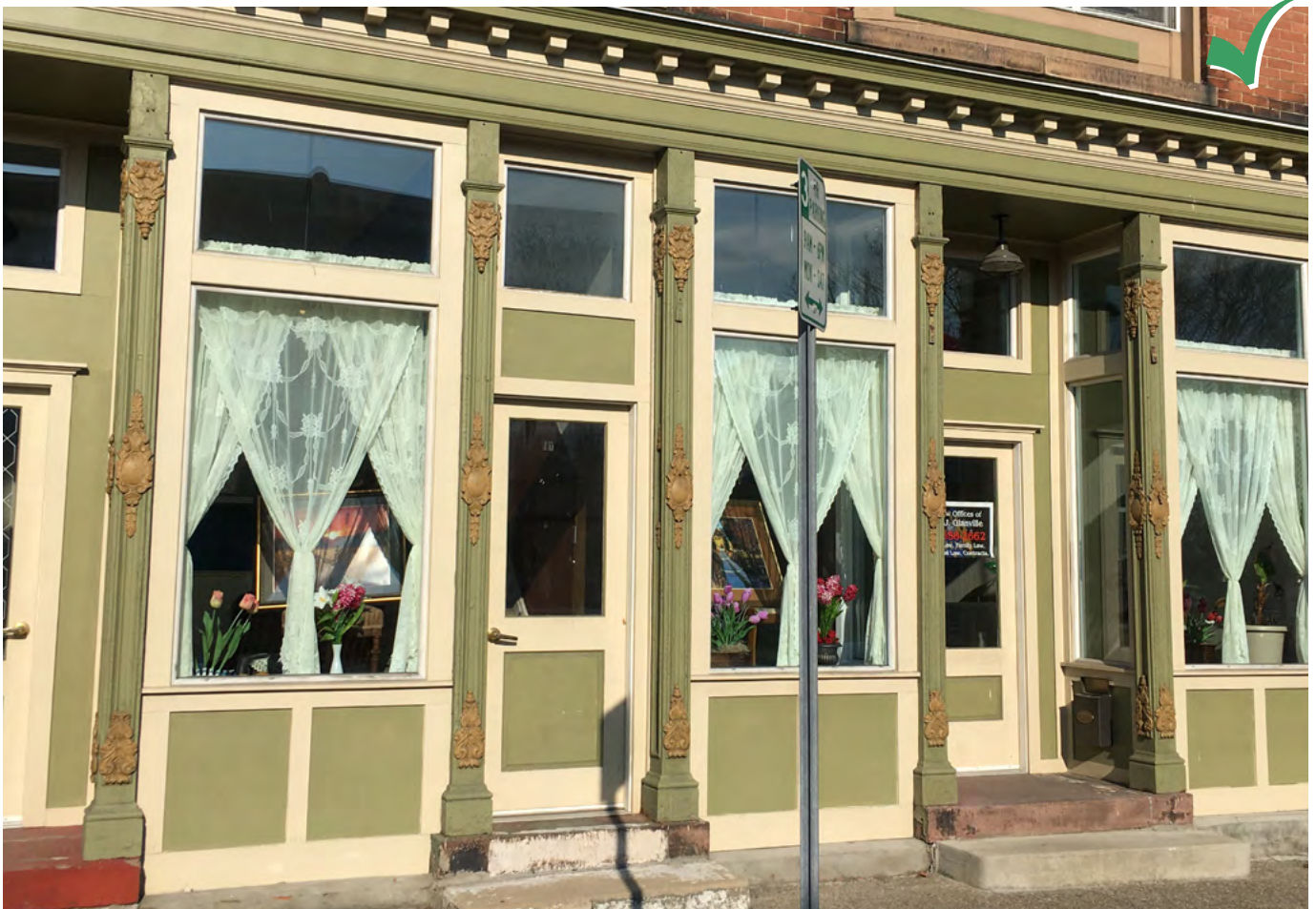
Use materials that can be repaired and maintained similarly to the original - such as fiber cement in place of wood.
