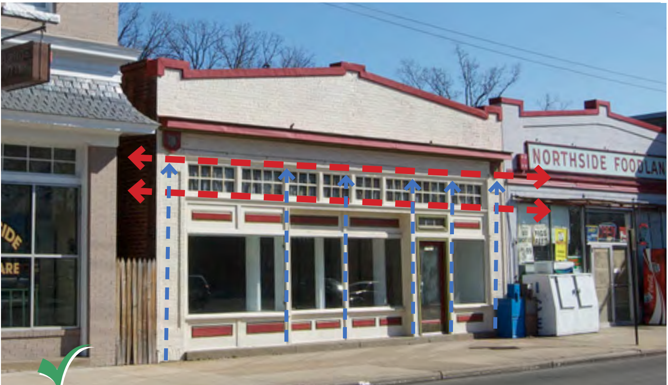
Use transom windows to add horizontal lines that break up the height of window openings. Establish a rhythmic pattern to break up storefronts with horizontal and vertical patterns.
