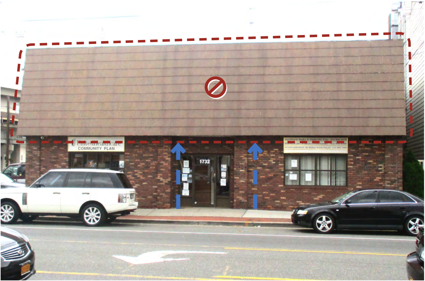
Avoid long, uninterrupted, plain surfaces that don't establish a rhythm. Do not interrupt an existing horizontal or vertical pattern.
