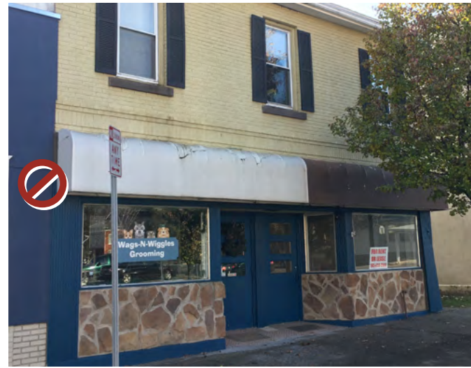
Don't use inauthentic materials on your storefront such as this stone veneer.
