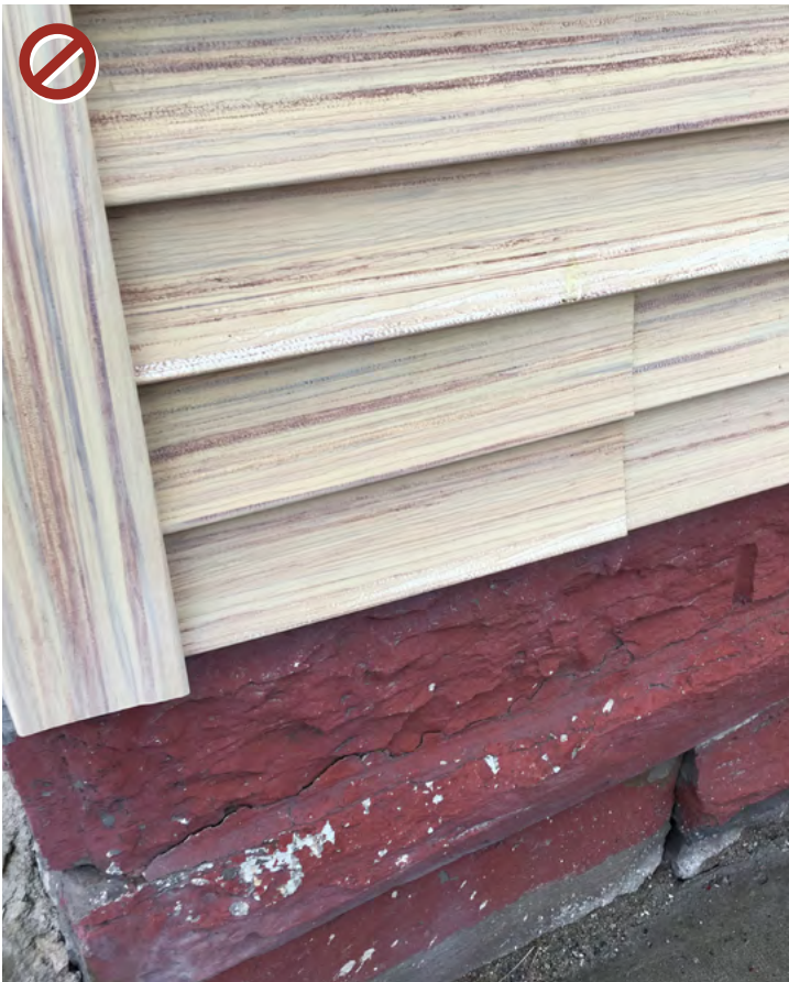
Do not use vinyl siding or paint a fake wood grain on it to simulate wood siding. Use fiber cement or similar.
