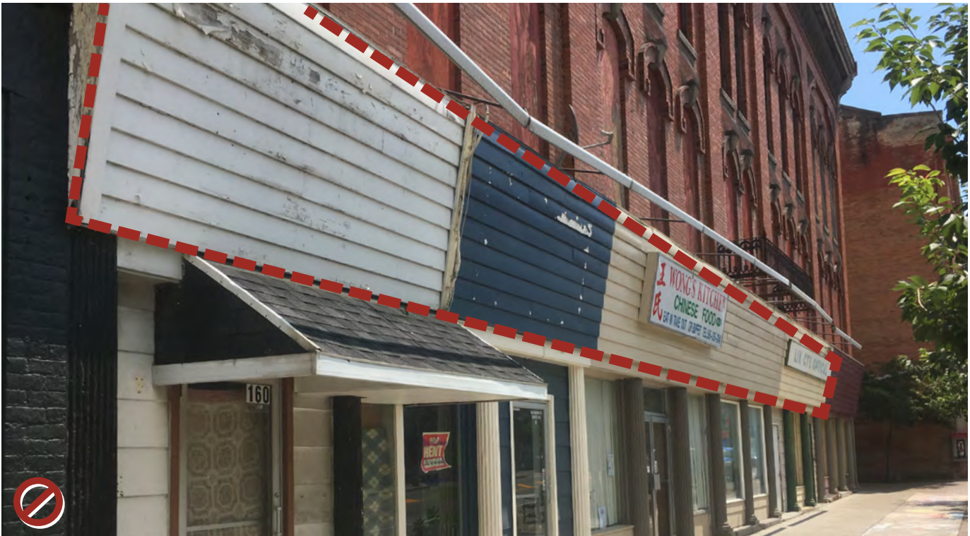
Do not cover original materials such as masonry or wood cladding with inappropriate materials such as stone veneers or vinyl siding. Do not cover up original storefront openings and details.
