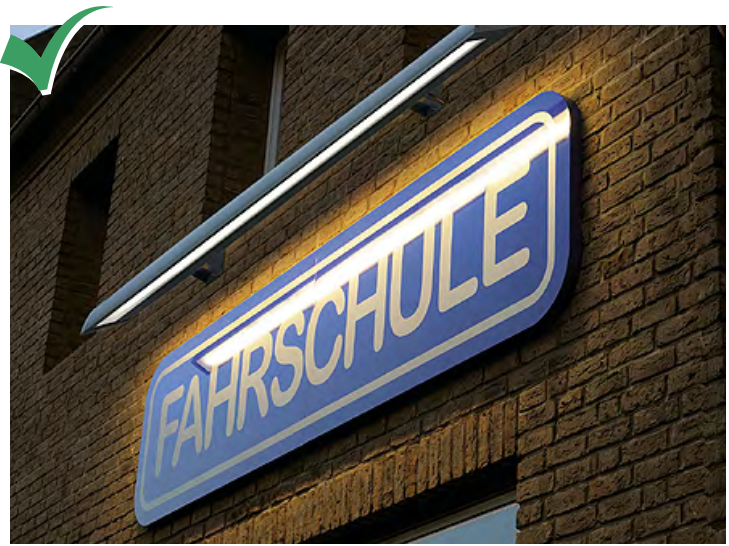
Use linear light fixtures for wall signs and other horizontal surfaces that need even lighting.
